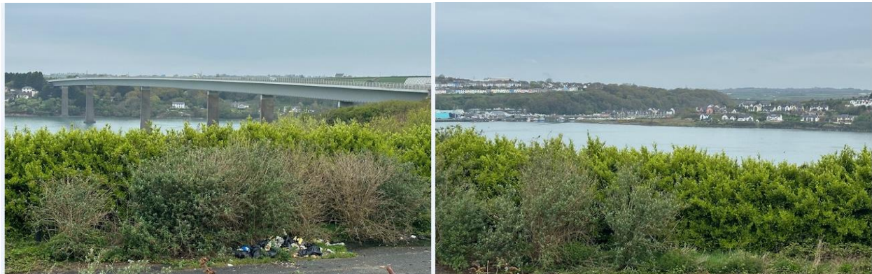
Views towards the Cleddau Bridge and the Estuary
