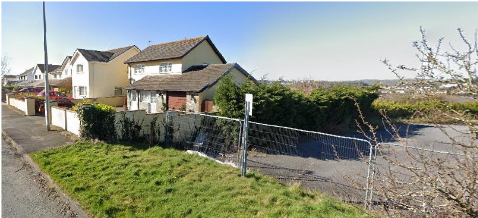
Side Elevation of No. 35 Essex Road
