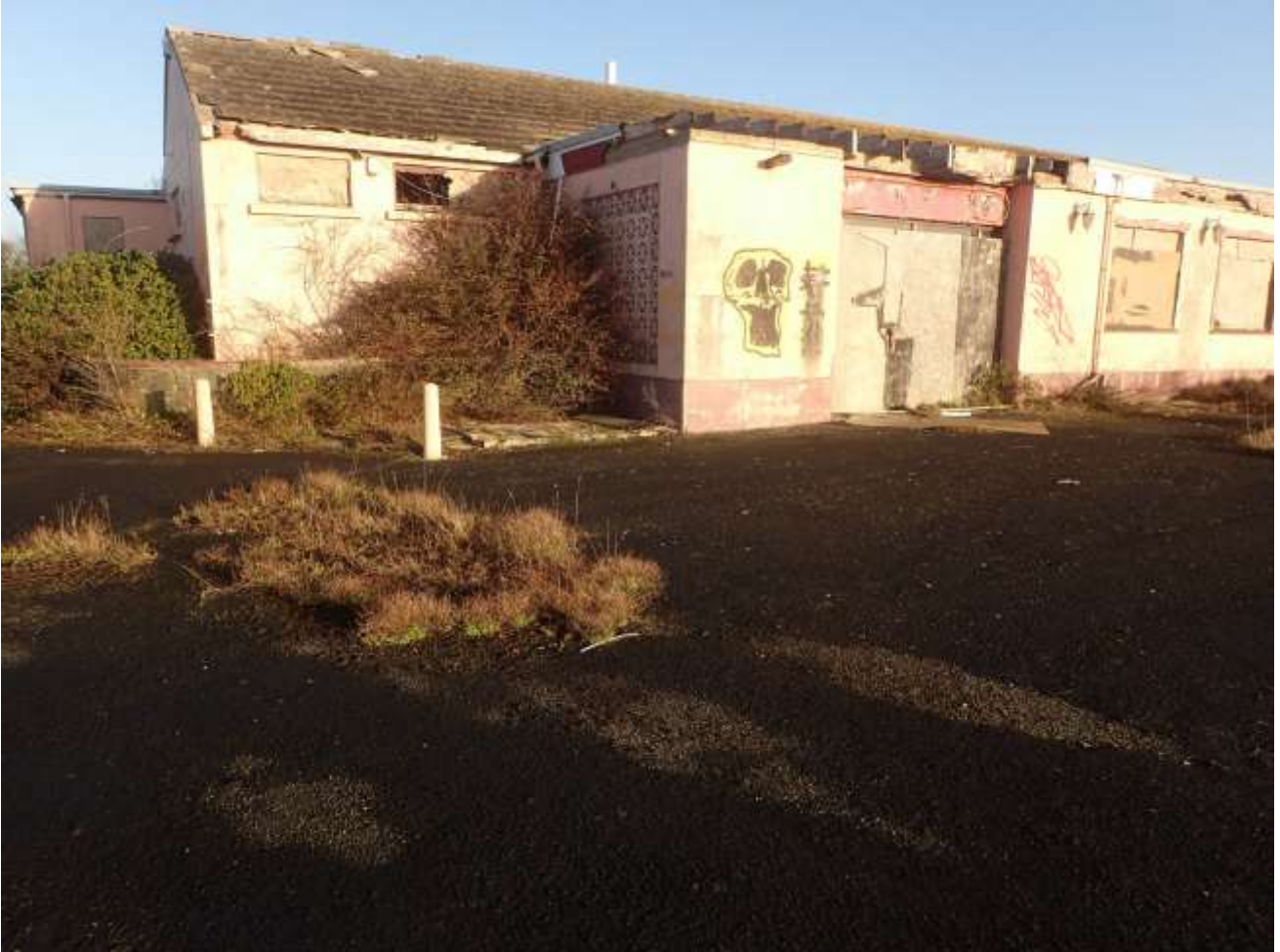
The former motel and associated hardstanding
