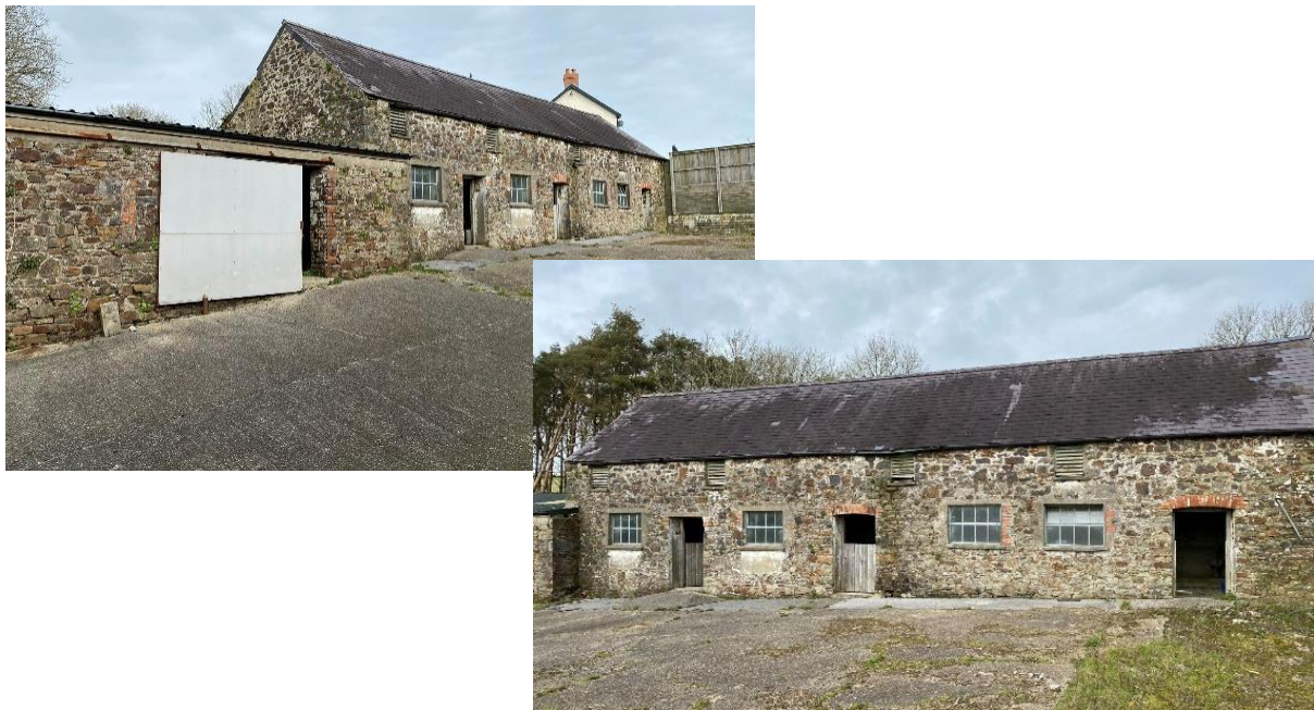
Existing Stone Outbuildings for Conversion
