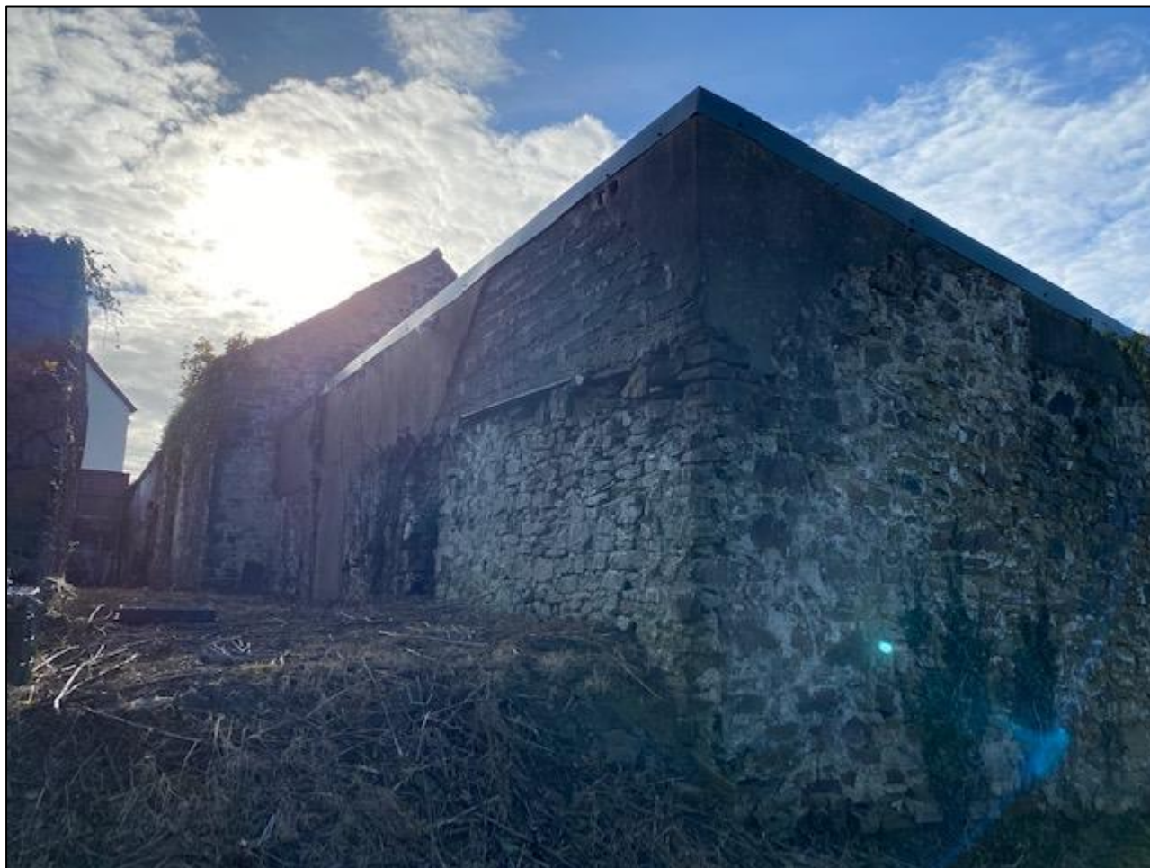
Figure 3. North eastern elevation of the barn.
