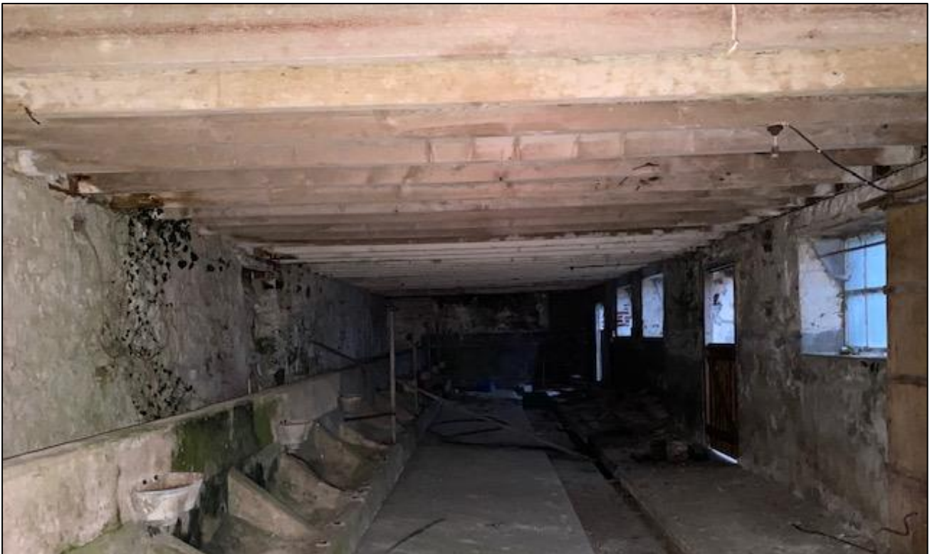
Figure 2. Internal view of the ground floor
