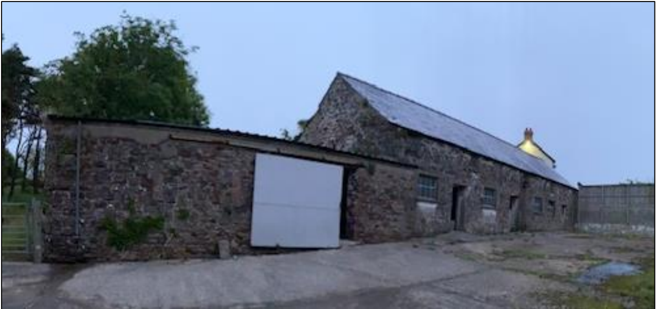
Figure 1. Northern and western elevations of the barn.
