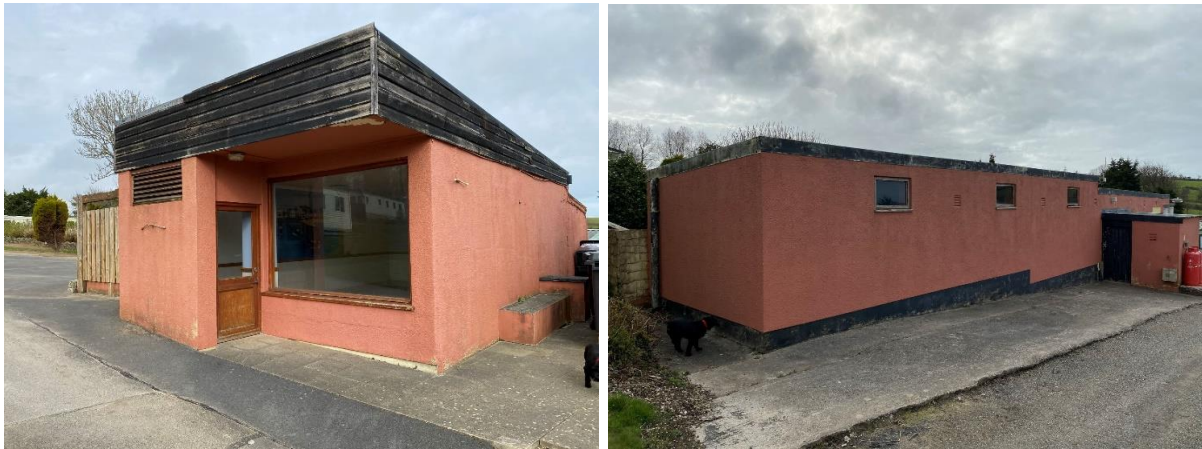
Pictures showing existing Amusement Room / Launderette / Diner to be demolished
