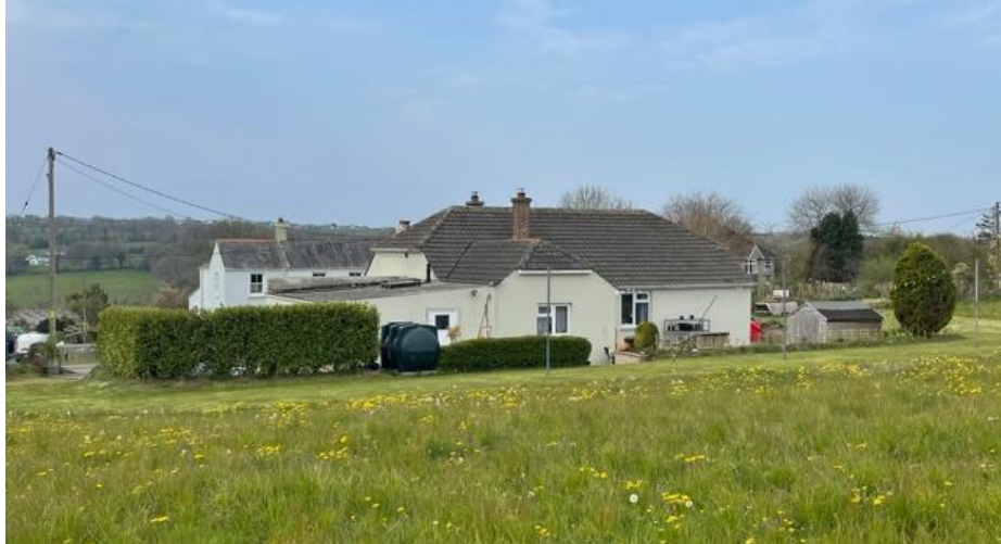
View of adjacent property 'Lyncroft'
